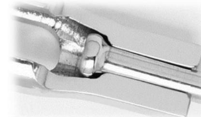
If any are found to be worn, or cracked, the rod must be re-headed. That doesn't necessarily mean the entire rod section needs to be replaced. If there is enough throw on the turnbuckle, then the rod in that section can be re-used. The rod will typically last significantly longer than the cold heads at the ends.
