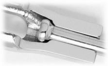
If any are found to be worn, or cracked, the rod must be re-headed. That doesn't necessarily mean the entire rod section needs to be replaced. If there is enough throw on the turnbuckle, then the rod in that section can be re-used. The rod will typically last significantly longer than the cold heads at the ends.
